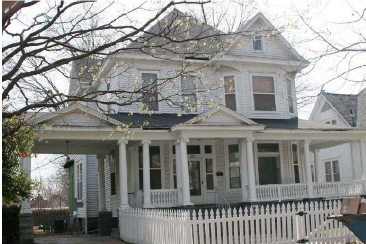
Figure 17. 507 South Sergeant Avenue, #113, 2011. Source: Historic/Architectural Survey of the Murphysburg Residential Neighborhood, Taylor & Taylor Associates, Inc.
